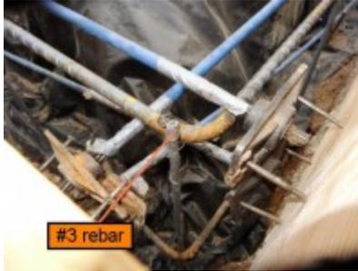
3. Another common issue with the installation of your home's foundation is standing water and poor grading and drainage. Grading is typically done by builders after the foundation has been poured, and sometimes later. This directs any recent rainfall into the foundation beams. This will significantly reduce the strength of the concrete when it mixes with the water, and should be avoided.
